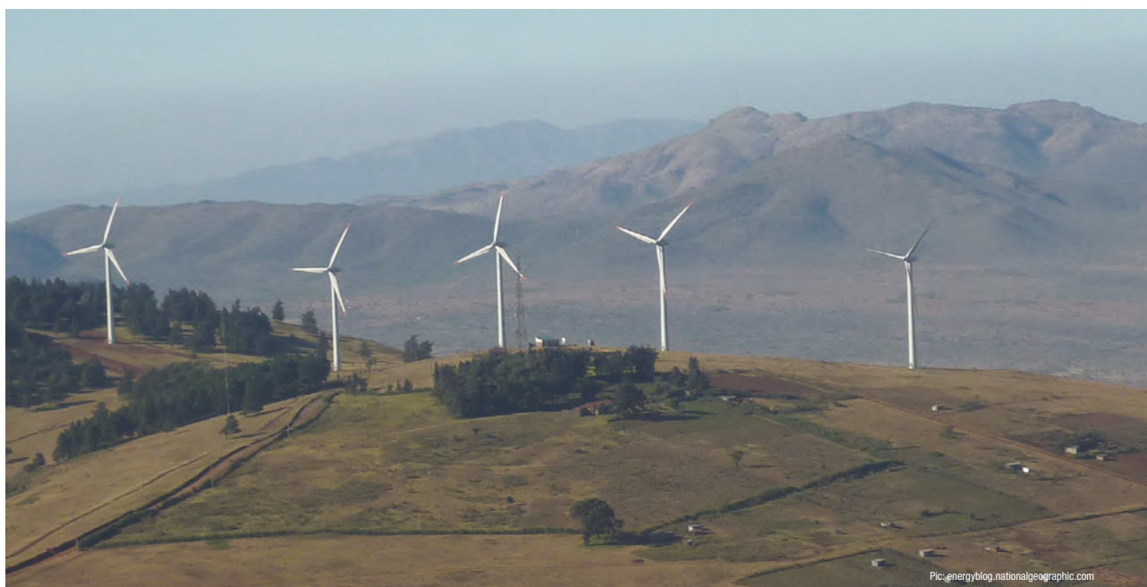
Ngong Hills wind farm
